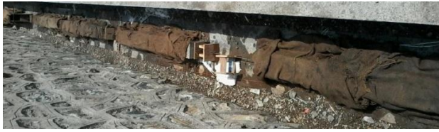
Fig.6 Curing of concrete blocks & beams
